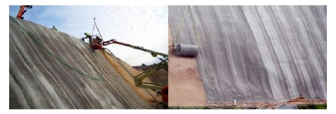
c) **Remediation**: Concrete weavers can be used to rapidly reline and refurbish existing concrete structures suffering from degradation and cracking.
