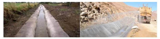
b) Erosion Protection: Concrete weavers can be used for slope protection as an easy and less expensive alternative for classic concrete structures. Becomes hard after hydration but still has some flexibility to prevent the concrete from cracking. Mostly used for protection against mud slides and rocks falling down the slope.
